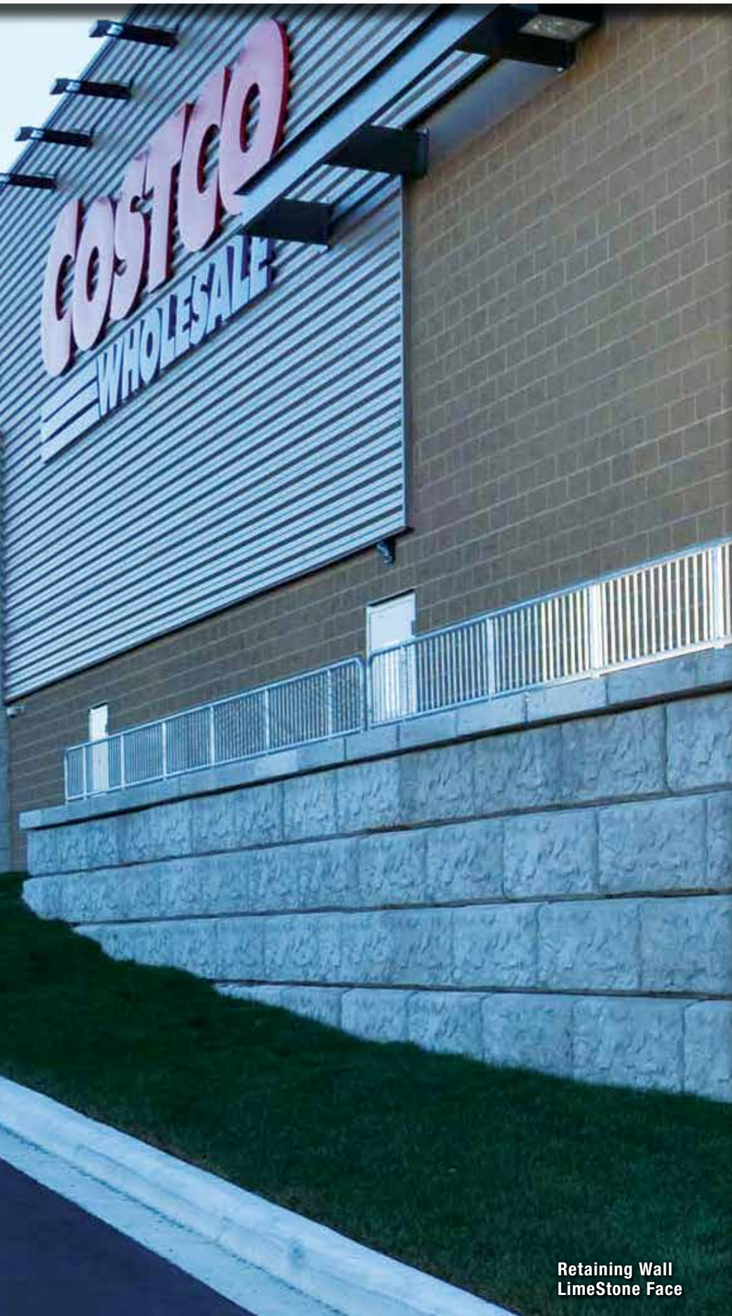
Retaining Wall LimeStone Face
