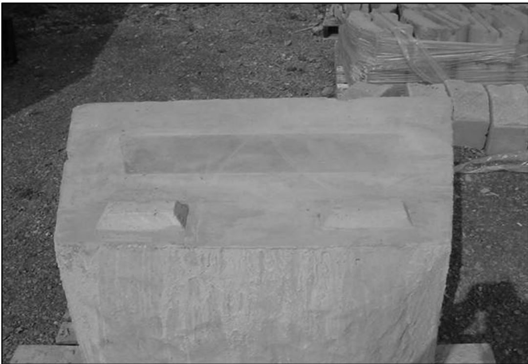
Figure 3: Photograph of the bottom of the London Boulder block showing the concrete filled section
